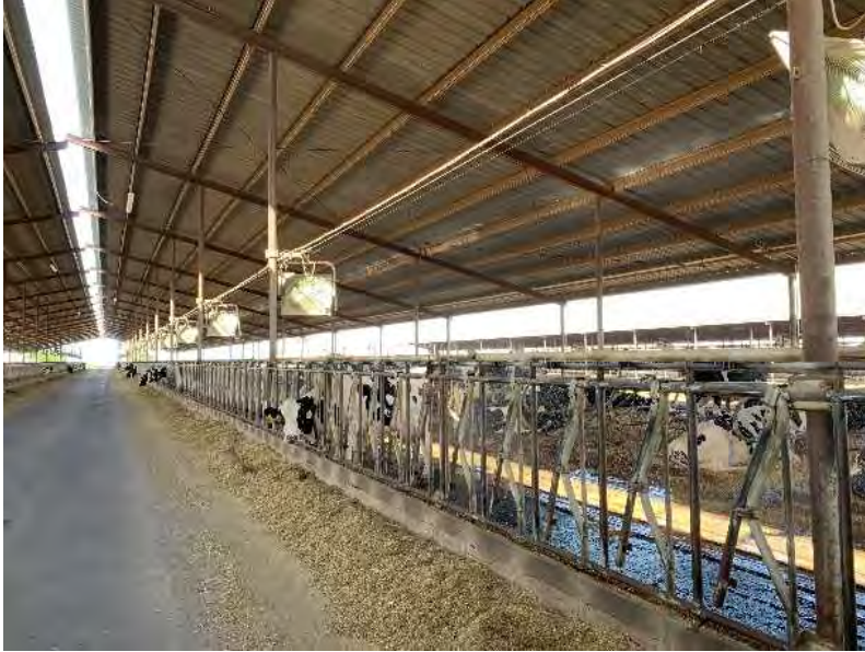
Picture 2. Fans and soakers placed together at the feed line are more efficient than either alone, reducing the need for excessive soaking overall. (Source: Grazyne Tresoldi)
